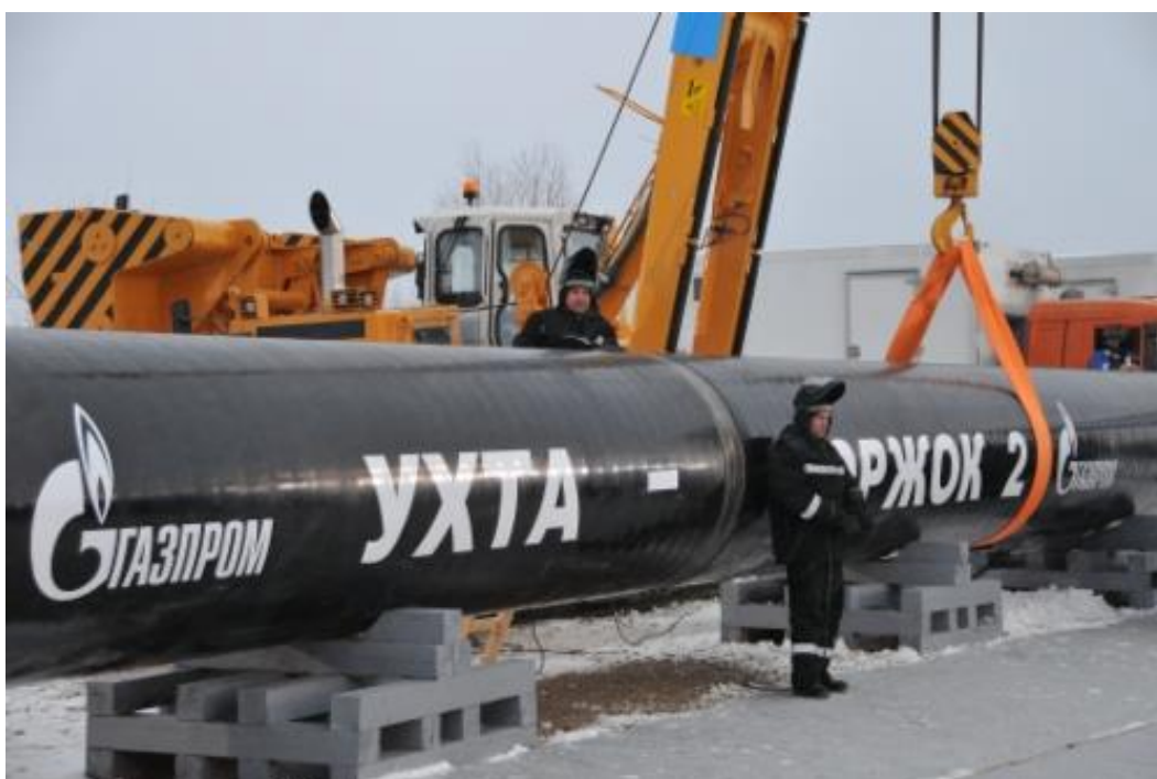
Figure 4-7: Construction of a onshore pipeline (Gazprom, 2016)
