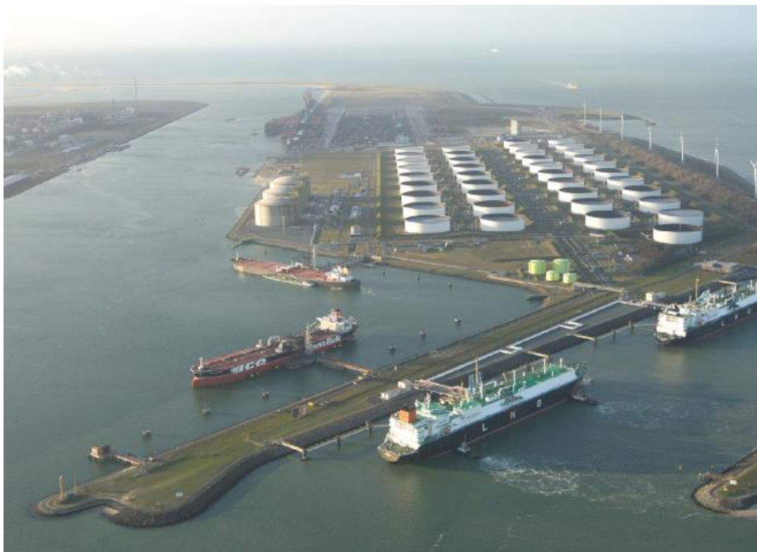
Figure 4-23: Example for a LNG import terminal (Regasification in Rotterdam, Netherlands) (King&Spalding, 2015)
