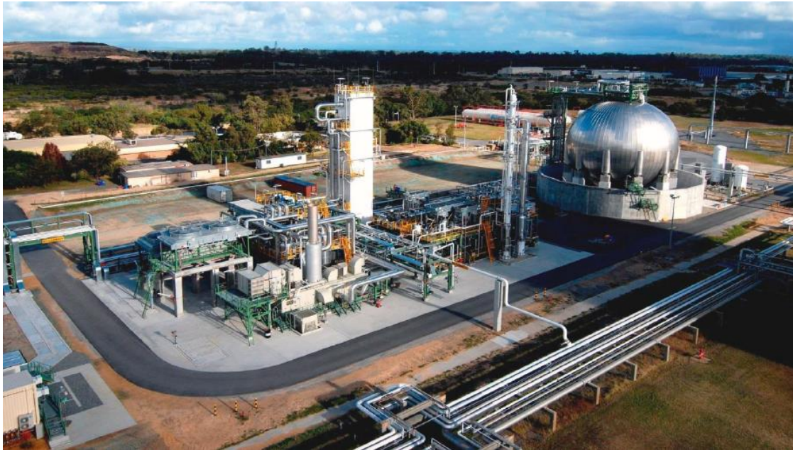
Figure 4-24: Example for a small-scale LNG plant (Liquefaction in Australia, under 1 MPTA) (IGU, 2016)
